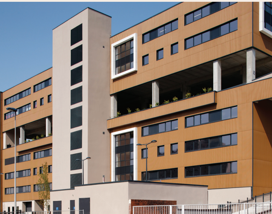
EcoCity Parc - Colombes (92) - CLAD 4 - Sun-tint • Architect: MW Architecture • © Fotocredits: Daniel Moulinet
