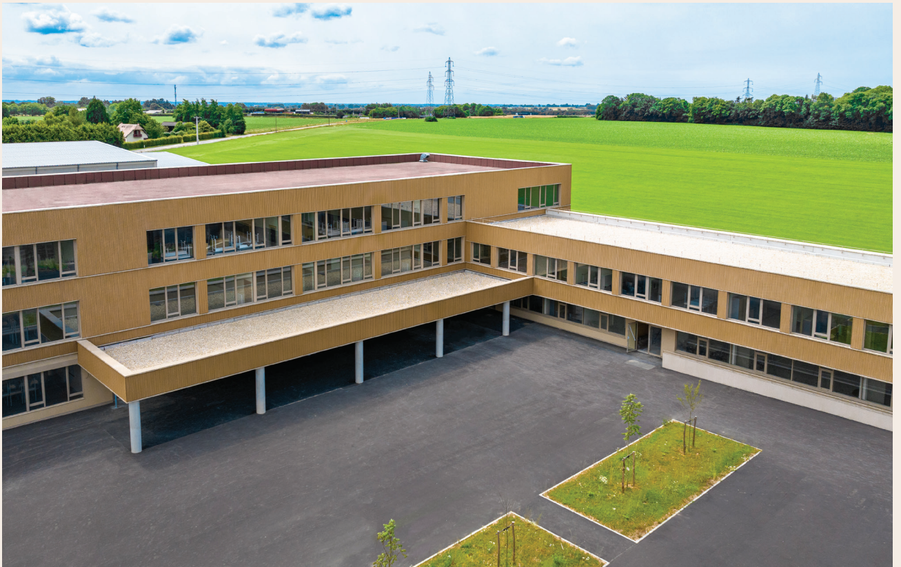
College Louise Michel - Bourneville (27) - COVER 6 - Sun-tint • Architect: ACAU & AP-MA • © Fotocredits: Initial Ingénierie - Matthieu Lecouvey
